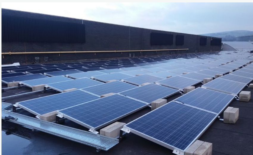
Macclesfield solar panels
